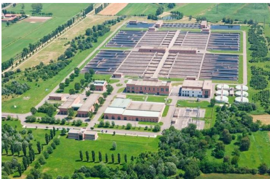
Figure 5 - View of the Nosedo wastewater treatment plant.
