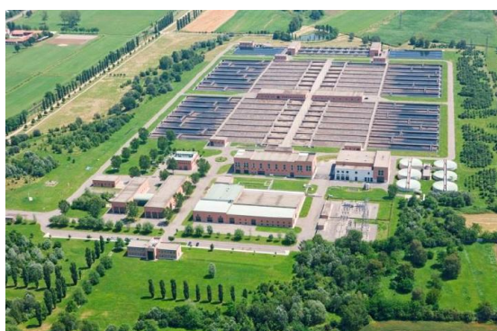
Figure 5 - View of the Nosedo wastewater treatment plant.
