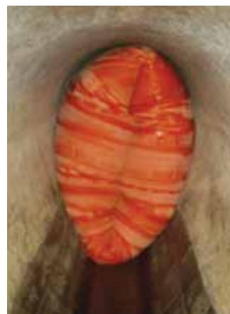
Cured In Place Pipe
