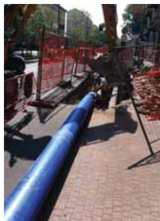
Slip Lining DN 400
