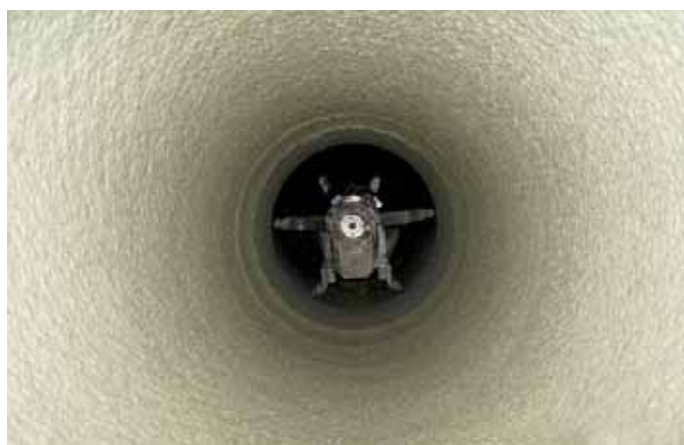
Cement Mortar Lining DN 1000
