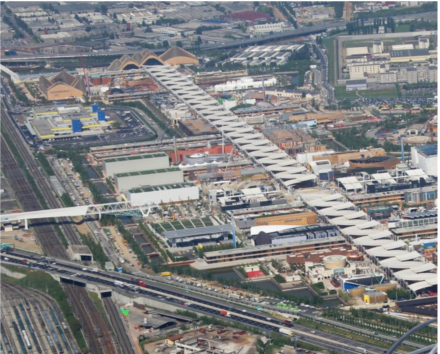
15 AREAL VIEW OF DECUMANO AND EXPO CENTER
