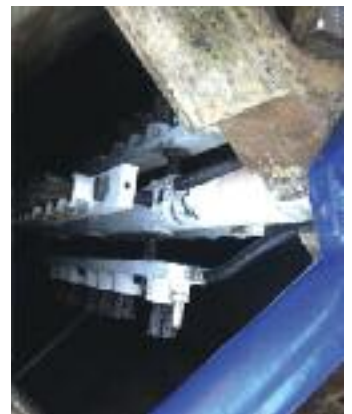
Extraction well maintenance
